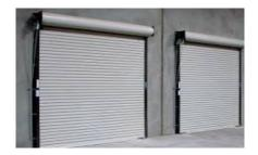
A Rolling Steel Coiling Overhead Door is a metal slatted door that rolls up above the dock opening.
